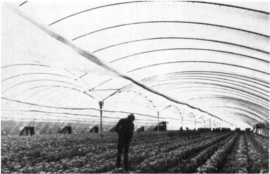
FIGURE 15 Air-supported structure of transparent plastic strips fastened to primary cables attached to secondary cables anchored to ground. (Goodyear)
