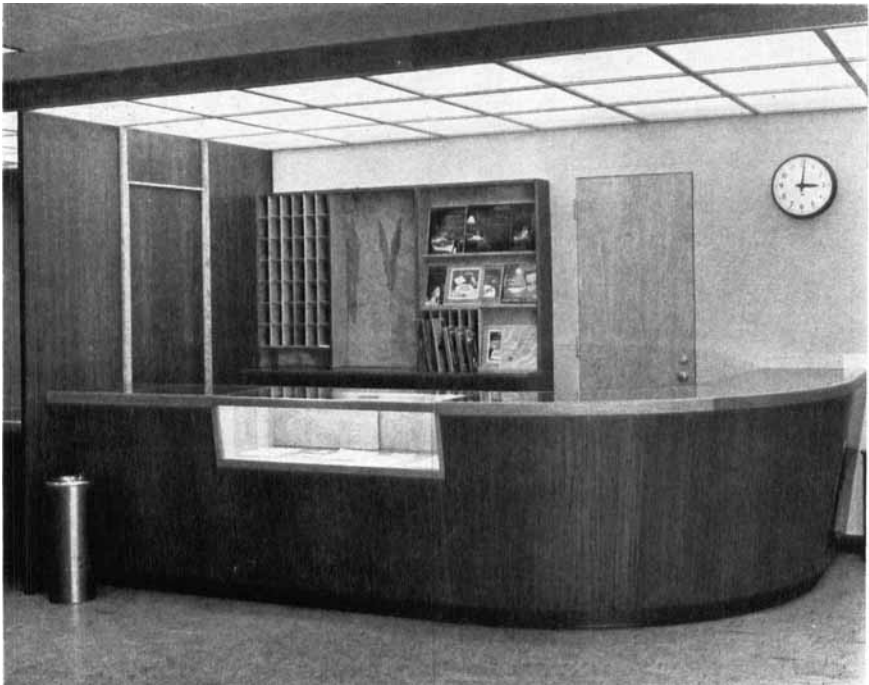
FIGURE 4 Luminous ceiling of lightweight panels. Counterfront and wall surfacing of high pressure decorative laminates. (Parkwood)
