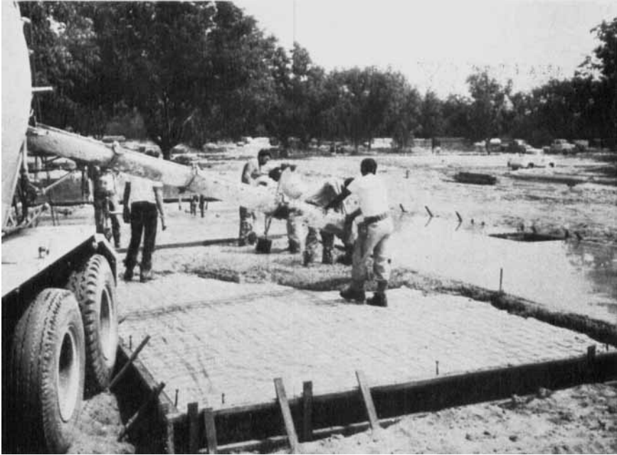
FIGURE 6 Polyethylene vapor barrier under concrete slab. (Union Carbide)
