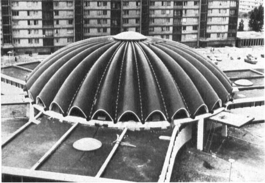
FIGURE 7 Market building roof of glass fiber reinforced polyester curved conoids, Argenteuil, France. (Stephane du Chateau)
